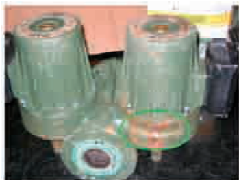
DMH 60/280-50T leakage zone
