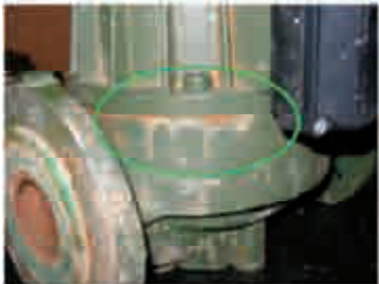
Leakage zone on BPH 120/280-50T
