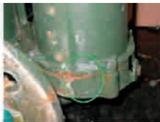
Leakage from condensate drain
