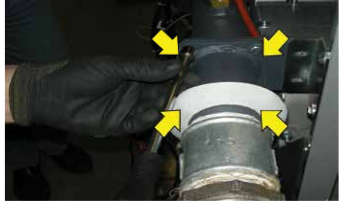
- Remove the four screws with a 10 mm socket wrench, then the gas flange
