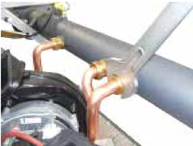
- Remove the gas fittings from the gas manifold using the 36 mm flat spanner.
