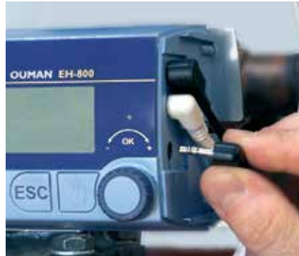
Detach the control knob from the valve and put the mounting kit into place. Press EH-800 into place, connect the sensors, plug it in and the unit is ready to use!
